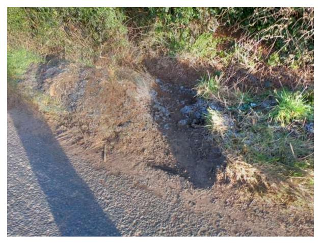
Grips cut at an angle are more likely to encourage water to flow from the road into the ditch. However, the uphill edge is still shaped to discourage this. The depth of the grip is better sitting well below the road surface.
