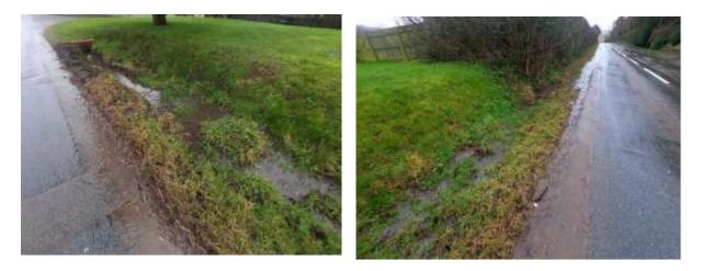
This is an example of where a roadside ditch is needed to clear the road. It is not a landowner issue. The damage that is being done to the carriage way is immense and the small cost of digging a roadside ditch would be insignificant compared to the costs of repairing the already damaged road surface. Edge erosion on this section is spectacular and up to 200 mm deep in places. A cyclist slipping into this trench could be seriously injured or killed.
