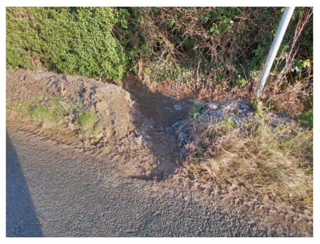
Grips cut in this way have limited ability to capture water flowing past them. Water will tend to run straight past. The grip is narrow, there is little clear definition of the side walls and spoil piled at the sides will simply wash back in. The bottom of the grip is only just below road level and will quickly silt up again.
