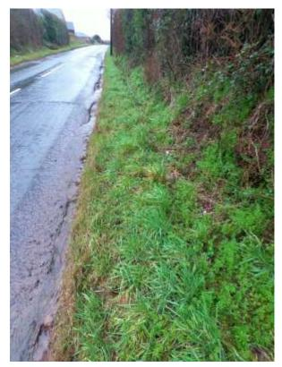
Below the farm there is evidence of ditches on both sides of the road, both of which were dry while water flooded down the road causing further edge erosion.
