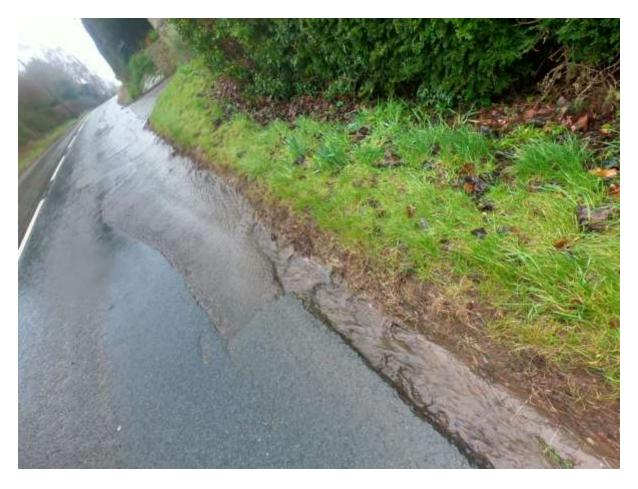
Just past Lower Ryland at the point where the road edge erosion starts there is clear evidence of a roadside ditch that is completely dry while the water ravages the road edge. This is not verge erosion, the carriageway is clearly damaged.
