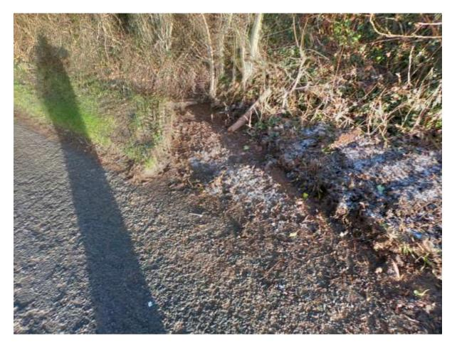
Of all the grips cut by BB on the B4221, this one stands out as being the best. Although it would benefit from a little more taken from the bottom, the sides are well defined, the lower face is at 45 degrees, and the upper face is cut back at a much more acute angle to encourage water to run off the road. The mouth at the roadside is much wider and the throat is at least 600 mm wide. This should be the standard for all grips.
