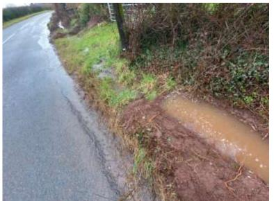
The sad thing about this is that all of the water in the ditch is as a result of the new grips successfully cut further up the hill. This blockage is spoiling all of the good work done further up. Again, water is flowing down here for the first time in years and the only thing preventing the water staying off the road is this single blocked culvert. A short blast with a jetting nozzle would resolve this issue and stop water from re-entering the carriageway.
