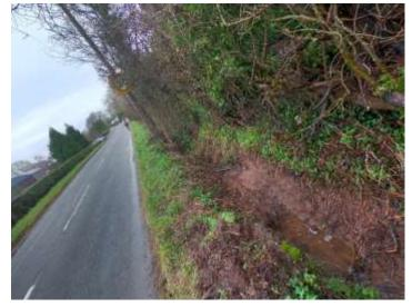
Water is currently coming through the culvert under the Chicory Crop entrance but is flooding out onto the road because of the blockage in the ditch. This is a perfect example of how digging grips is showing up the shortcomings in the ditch profile.
